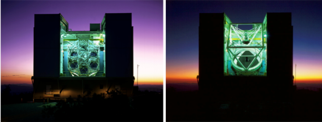
Figure 3.1: Left: Former MMT with six single 1.8 m mirrors. Right: Today's configuration with a 6.5 m mirror (MMTO 2022).
