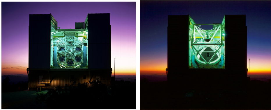
Figure 2.1: Left: MMT telescope with the six separate 1.8 m mirrors before the 6.5 m mirror upgrade Right: MMT telescope with on 6.5m Mirror, the current configuration.
